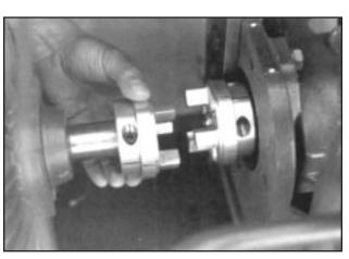
Install couplings on pump and motor shafts.
